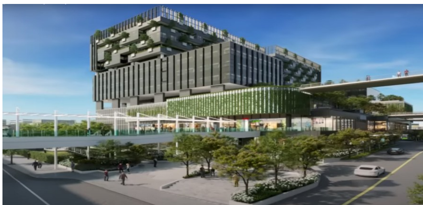
TRUE DIGITAL PARK BY WHIZDOM LANDMARK ( OFFICE BUILDING 12 FL. )
