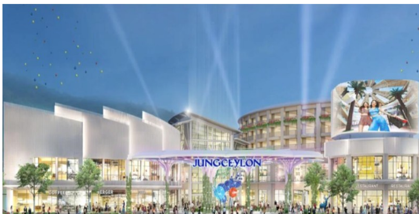
JUNGCEYLON PHUKET (RENOVATION)
